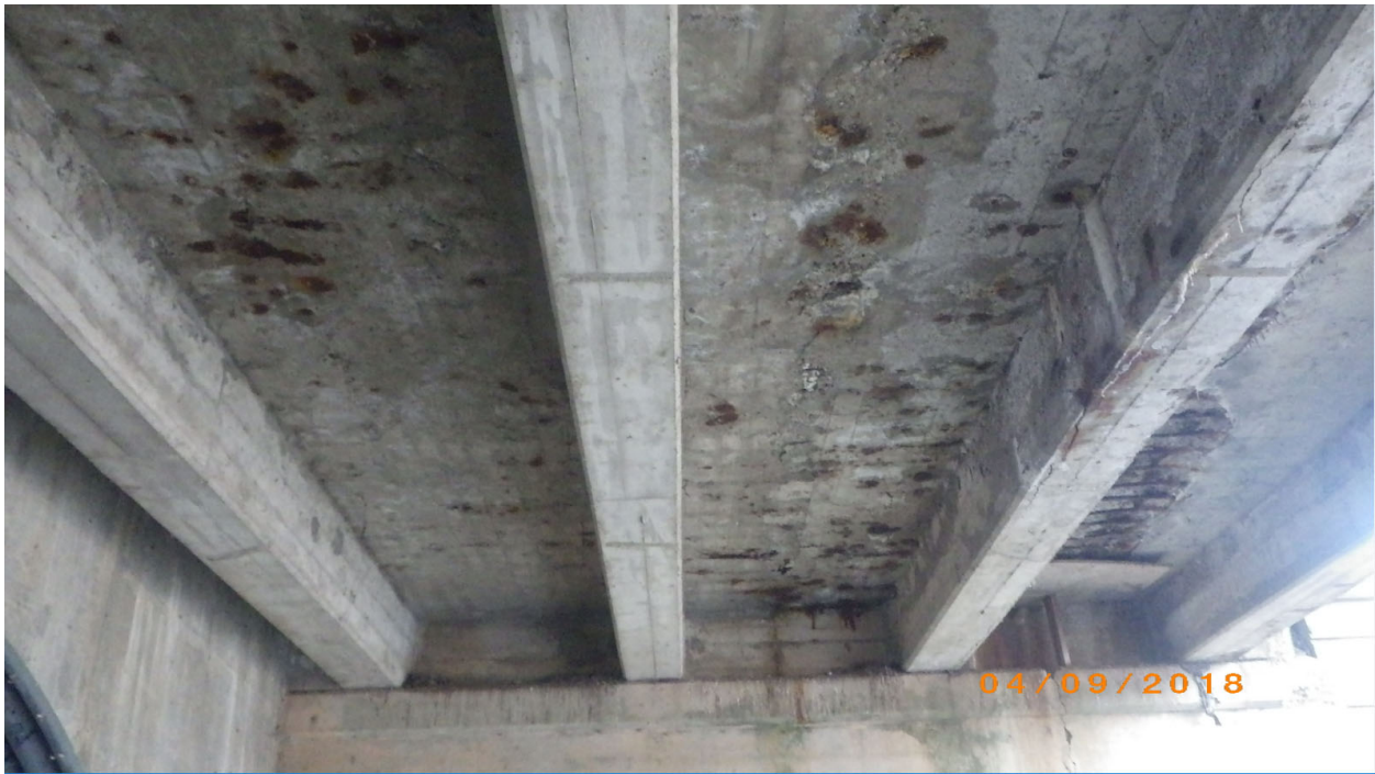
Picture 7: Rust Staining on underside of T-Beam deck
