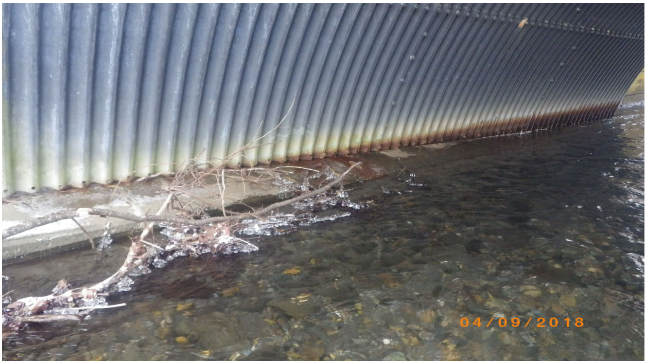
Picture 6: Rust Staining on metal pipe along water line
