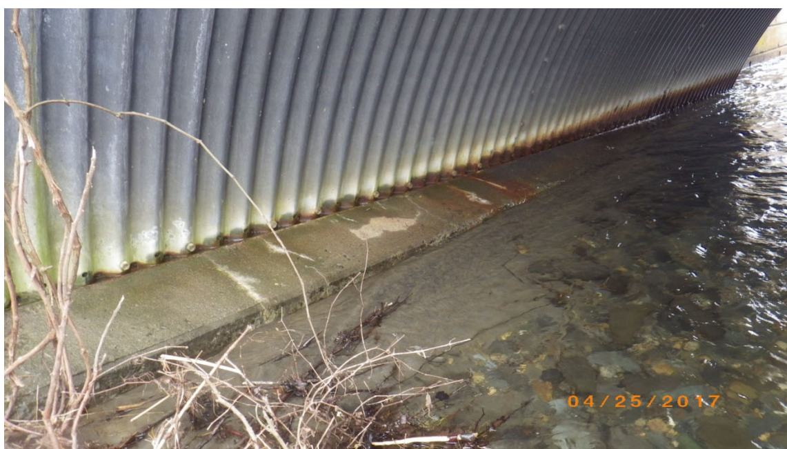
Figure 3.1: Cobbles within streambed and sediment deposition at abutment foundation of the pipe arch.
