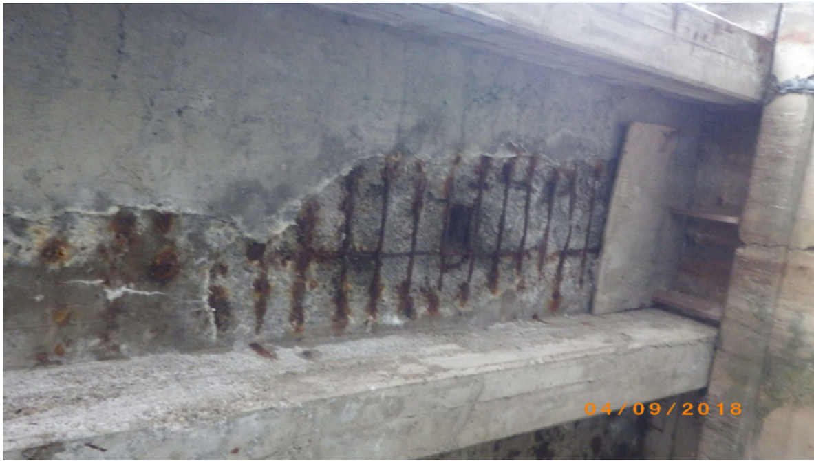
Picture 11: Deck Deterioration
